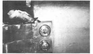
Close-up view of a defective 10,000 AMP bus connection. Note: Feeler gauge between mating surfaces.
