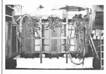
Failure of extra flexible, high voltage connections.
