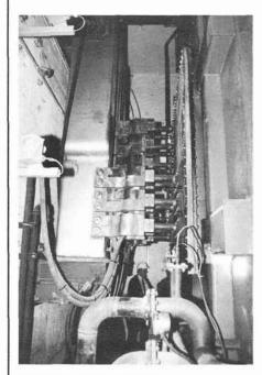
10,000 AMP Connections: Overheating on secondary (750V) side.
