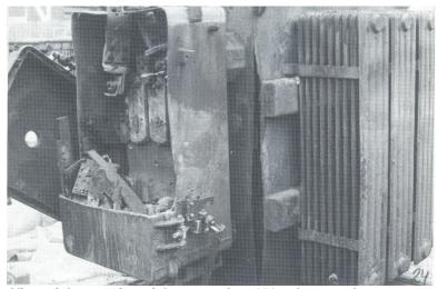
View of the remains of the secondary 600 volt network protector for the above transformer, damage due to sustained internal and external arcing and oil fire. Note: The split in the transformer tank, due to an internal fault, caused a fire and destroyed all electrical equipment in the vault.
