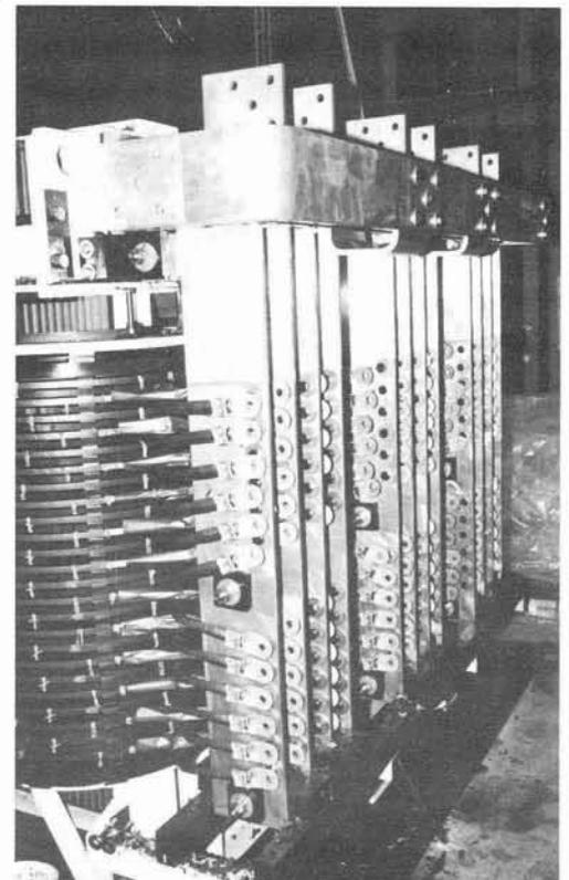
*Internal connection failure on 18 MVA transformer.*
