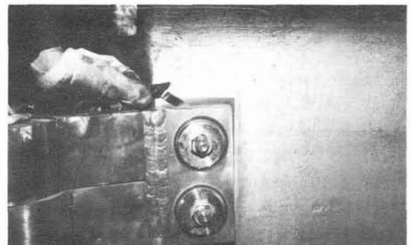
*Close-up view of a defective 10,000 AMP bus connection.
