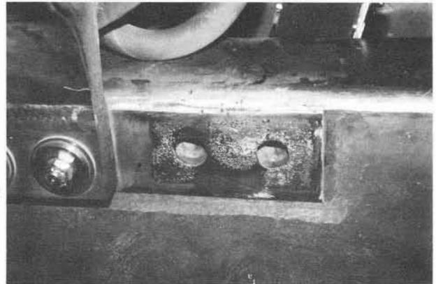
*Close-up view of deteriorated/overheated 10,000 AMP water-cooled connection.*
